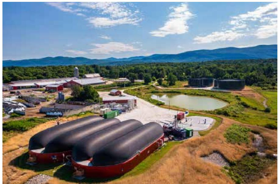
Vanguard Renewables uses anaerobic digesters on farms such as one in Vermont to produce renewable natural gas
